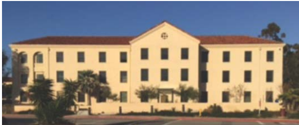
Newly refurbished Building 209 on the West L.A. VA Campus.
