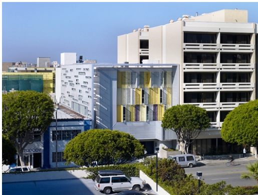
Step Up on 5th Santa Monica, California. Brooks + Scarpa Architects
